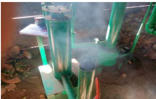
Gambar 6. Filter dan Gas cooler
